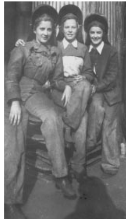
Lula Barber, Meta Kres, and Meda Brendall outside the welding shop at the Bethlehem-Fairfield Shipyards, Baltimore, Maryland, 1942. (VHP/Brendall/Coll. 4951)
