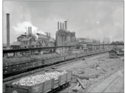
Illinois Steel Works, Joliet http://www.loc.gov/pictures/item/det1994004559/PP/
